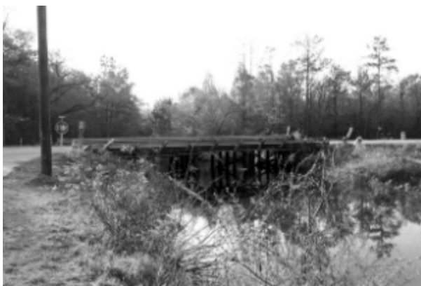
The bridge at French Quarter Creek. Brabant's Plantation and the historical marker are to the left
